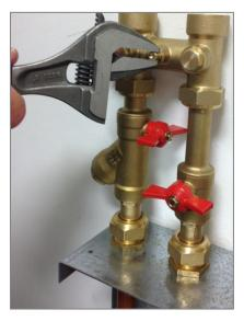
The whole primary system should be cleaned and flushed in accordance to BG29/2021 before filling ModuSat<sup>®</sup> heat interface unit.
