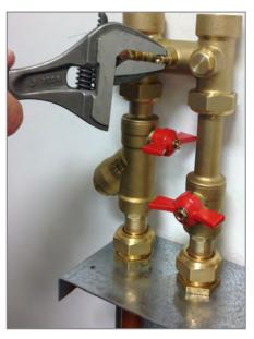
When the unit is installed and the primary network is cleaned or flushed, the valve kit should be used to ensure the unit is bypassed while cleaning or flushing the system.
